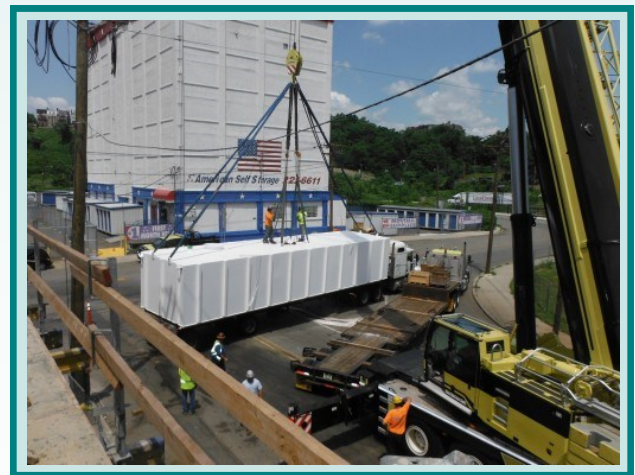
Sergio Borges —“For this multi-unit building, we are rigging to the second floor, a required secondary water supply tank. The tank is designed to supply 22,500 gallons of fire protection water.”
